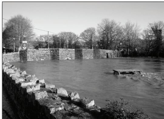
Lostwithiel Bridge in the flood of 17 November 2010.
